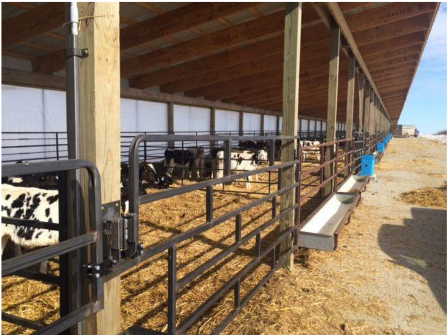
Fig. 7. A modified open front transition facility in South Dakota. Note the waterers are on the outside of each 10 head pen. This keeps water contamination of the pens on hot days to a minimum.
