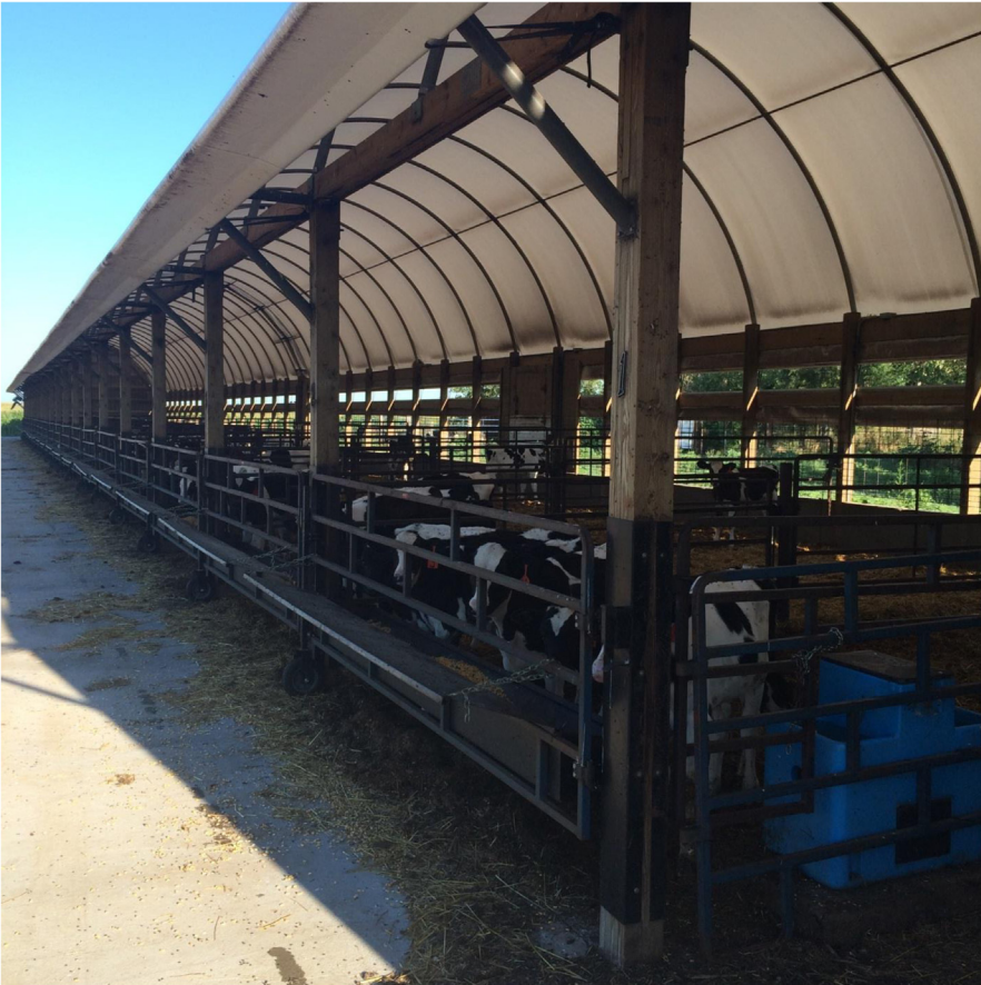
Fig. 5. A hoop structure transition facility in South Dakota. Note polylined protected feed bunks. Waterers inside each 10 head pens do result in water contamination of the pens on hot days when calves flutter the water out of the waterers into the bedded pen areas.
